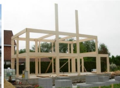
Paal en balk methode (Bron: natural build )
