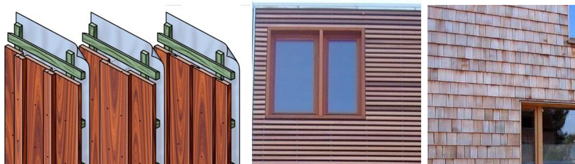
Verticale beplanking, illustraties sbrcurnet.nl
